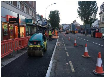
Bomax Scan Kerb was chosen for the project, due to the product availability with substantial UK stock holding, the speed an ease of installation, a no dig solution ruling out the risk of service strike, and with no material to cart away, the stick down kerbing solution saved many hours on installation time, cut down on the noise and dust pollution and reduced the amount of traffic disruption through the installation period, the overall finished appearance looks like a traditional kerb run
